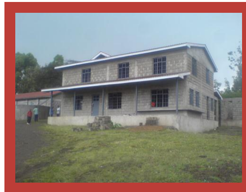
New Orphan Home at PCH under construction
