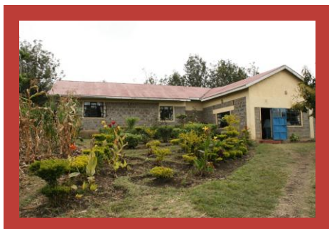
Current Orphan Home at PCH
